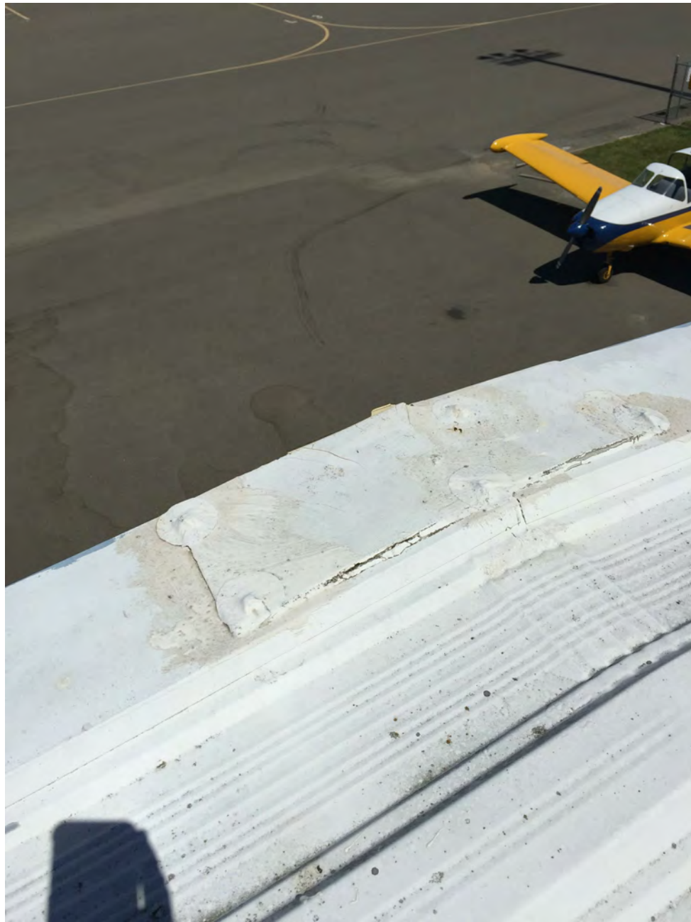
EXISTING ROOF FLASHING AT PEAK (NORTHWEST)
