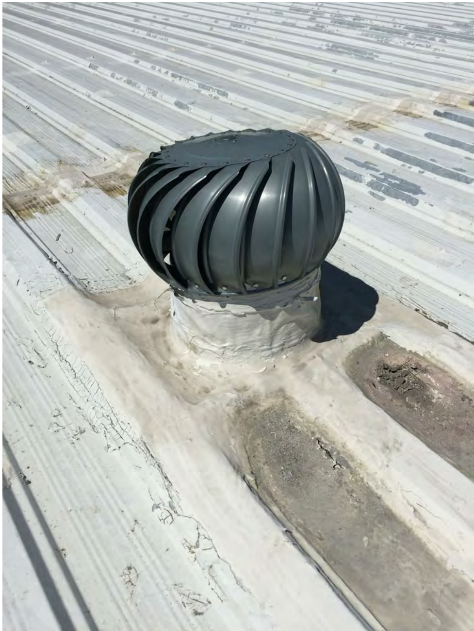
EXISTING TURBINE VENTILATOR, WOTH CAP AND FLASHING
