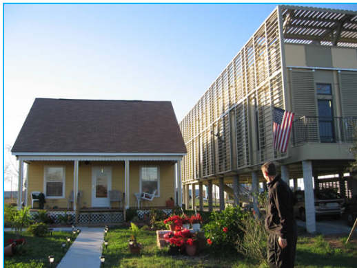
Figure 16. Old and New Homes in New Orleans.
