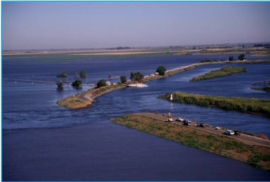
Figure 13. Aerial View of 2004 Levee Break at Jones Tract in the Delta
