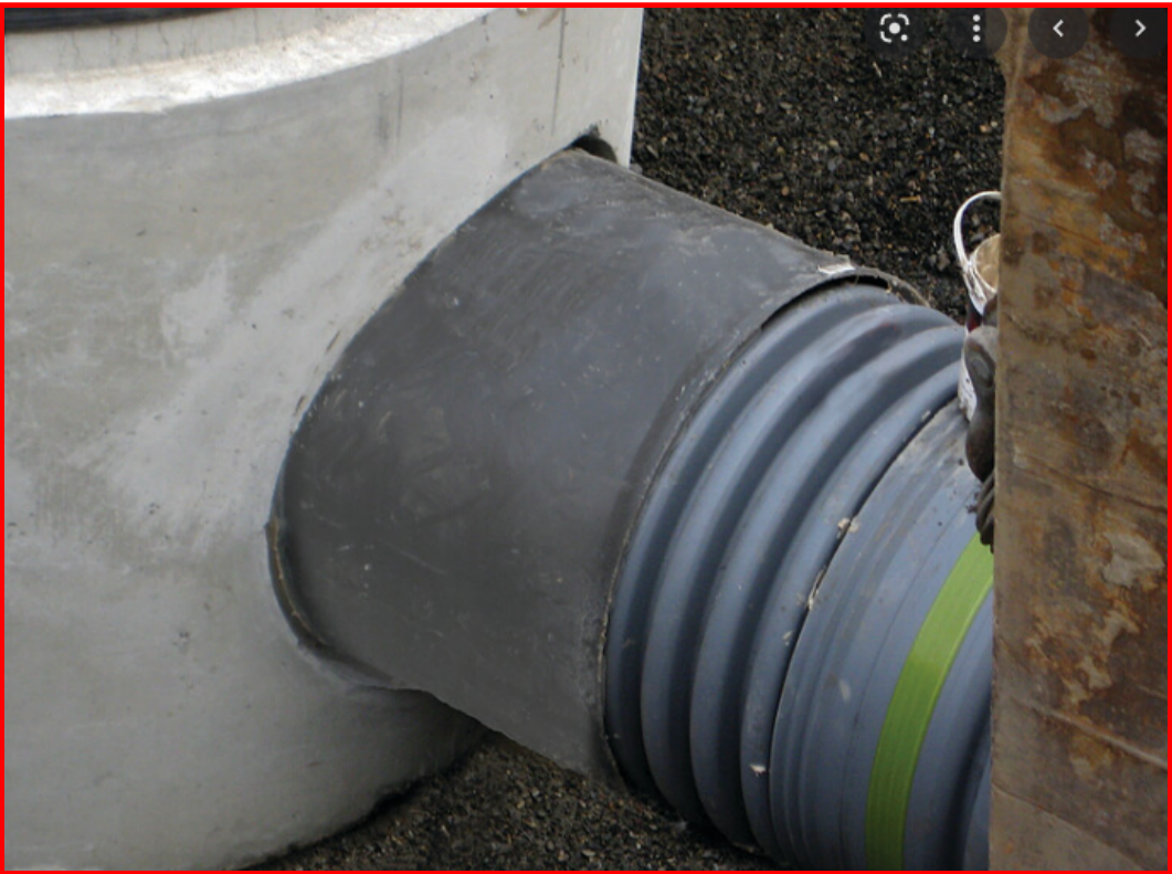
Knock a hole on the side of existing Drain Inlet and cement grout 4 inch corrugated pipe
