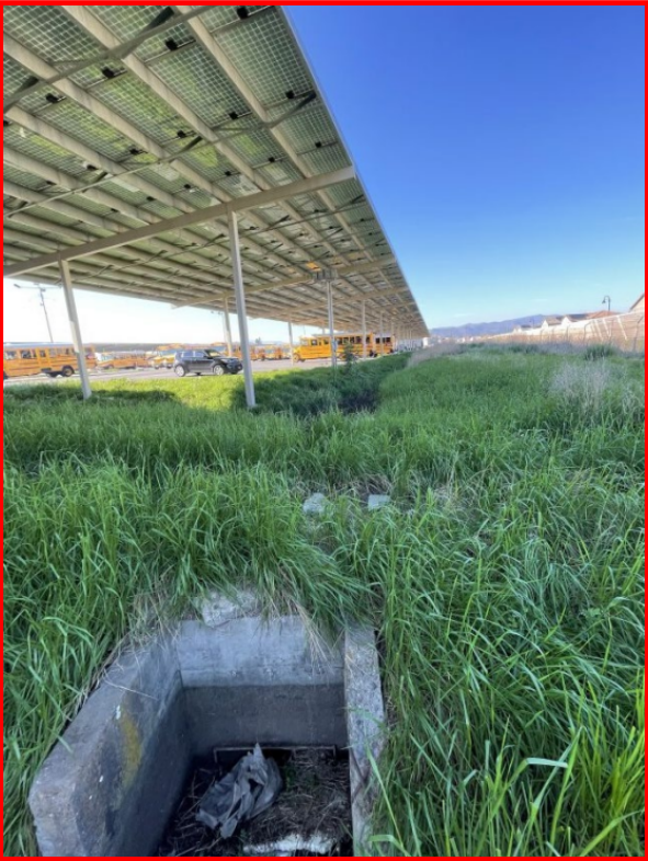
Clean out Existing Drain Inlet. Provide wattles for storm prevention pollution program
