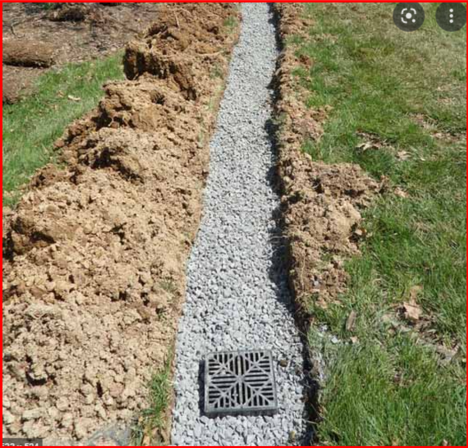
Backfill French Drain with 3/4 round Drain Rock Flush to Finish Grade
