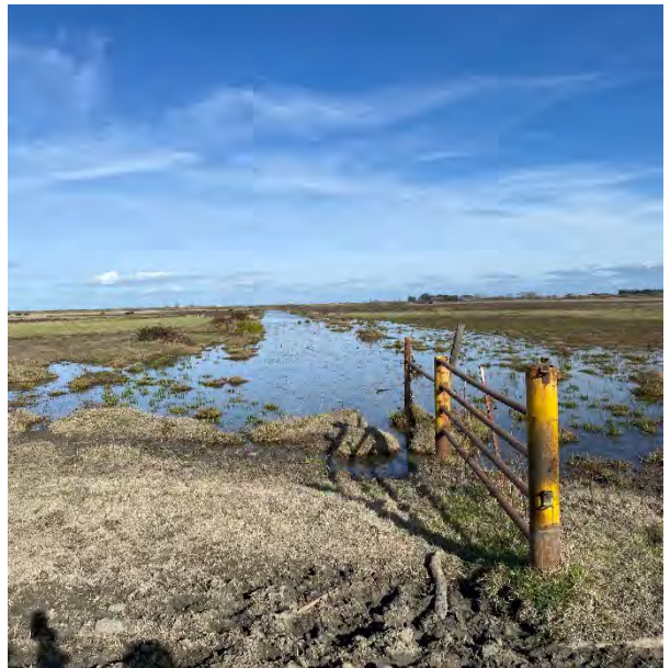
Photograph 4. Water spills from the central portion of the degraded berm to the northwest creating a human-made and managed emergent marsh and seasonal wetland.
